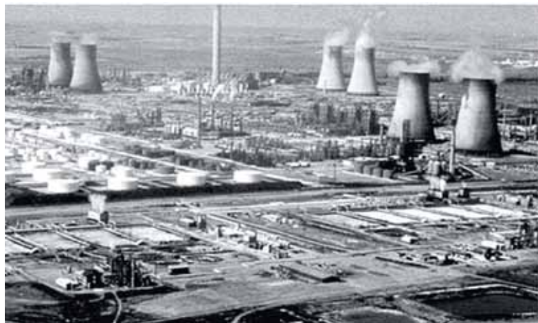
Sasol units II and III in Secunda, South Africa.
